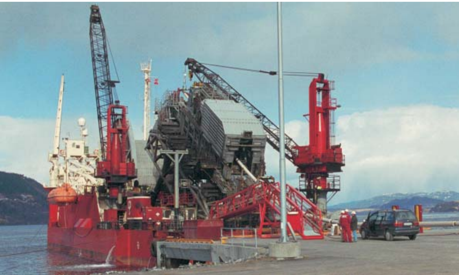
The Technip Offshore vessel "Apache" winding steel pipes at Orkanger.
