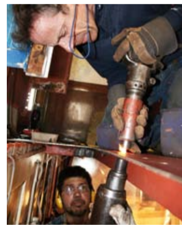
Once the rivet and the bucking bar are in place, a pneumatic hammer batters the rivet from above.
