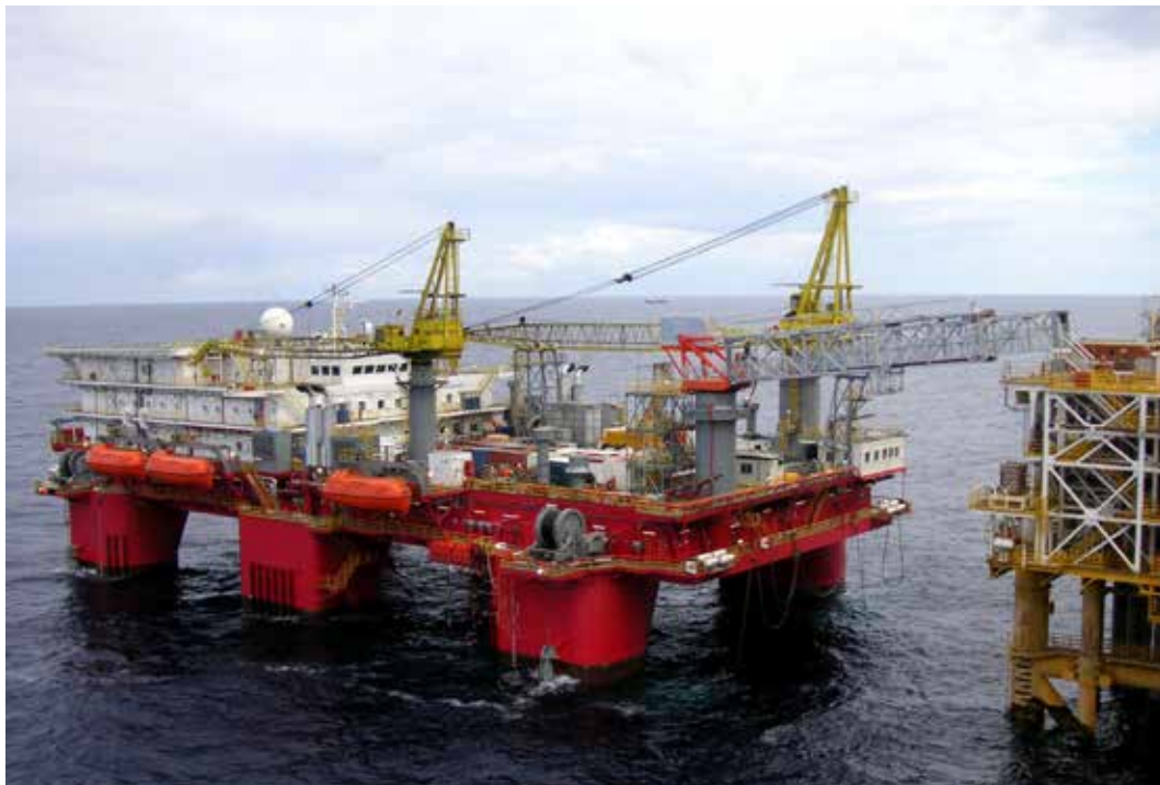
The 'Safe Concordia' accommodation and support platform. A mobile EFD Induction Minac system was used to pre-heat the weld area during the welding of a patch onto a crane tower.
